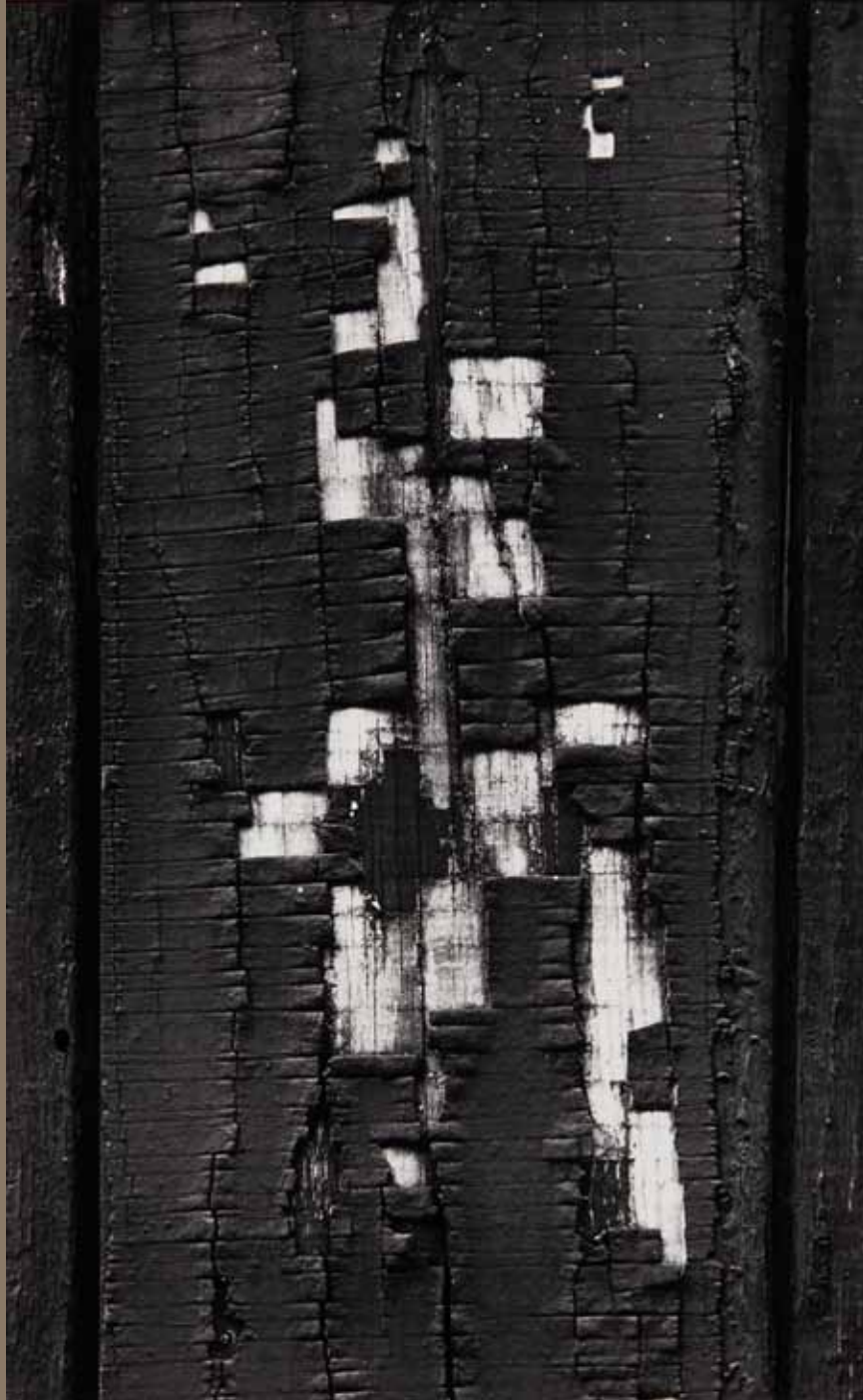
PEELING PAINT, BACK BAY, Boston, MA, 1956 19 x 11.5" PC186
